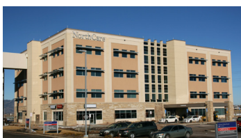
Northcare at St. Francis 6071 East Woodmen Road 11,956 SF For Lease (divisible)
