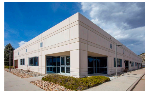
CENTENNIAL TECHNOLOGY CENTER 4920 Centennial Boulevard 59,970 SF for sale Stand alone single-story owner/user sale
