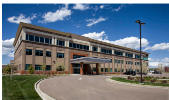
Briargate Medical Pavilion 4105 & 4125 Briargate Parkway 19,083 SF For Lease (divisible)
